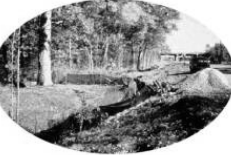
5. Erosion & Sediment Control
